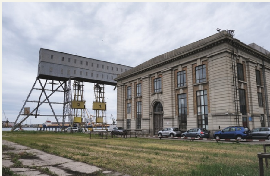
Power plant, Port of Constanta
